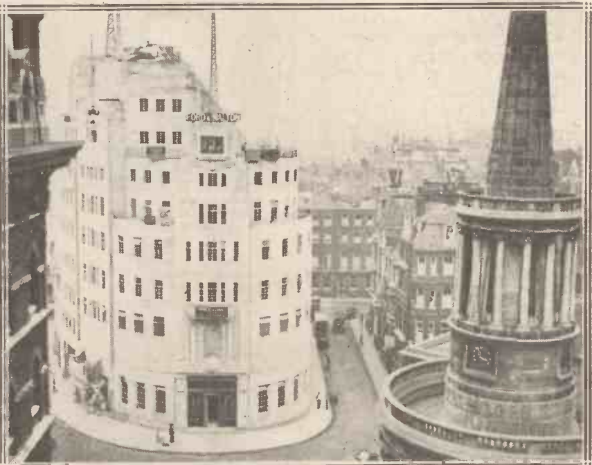
This is a view of the new Broadcasting House, London, W.1, which is equipped with twenty-two studios. How the programmes start and how they reach your aerial is told with concise clarity in the article that begins on this page.
