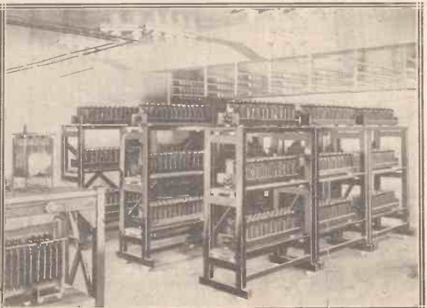
All the amplifiers are fed from accumulators, and over one mile of wire is necessary merely for the battery connections.
