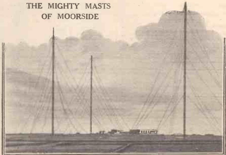
This is a view of the three 500-ft. masts of the new North Regional Station at Moorside Edge, near Huddersfield, Yorks. Look out for the tests from this—Britain's latest twin broadcast. (Wave-lengths, 479 and 301 metres.)
