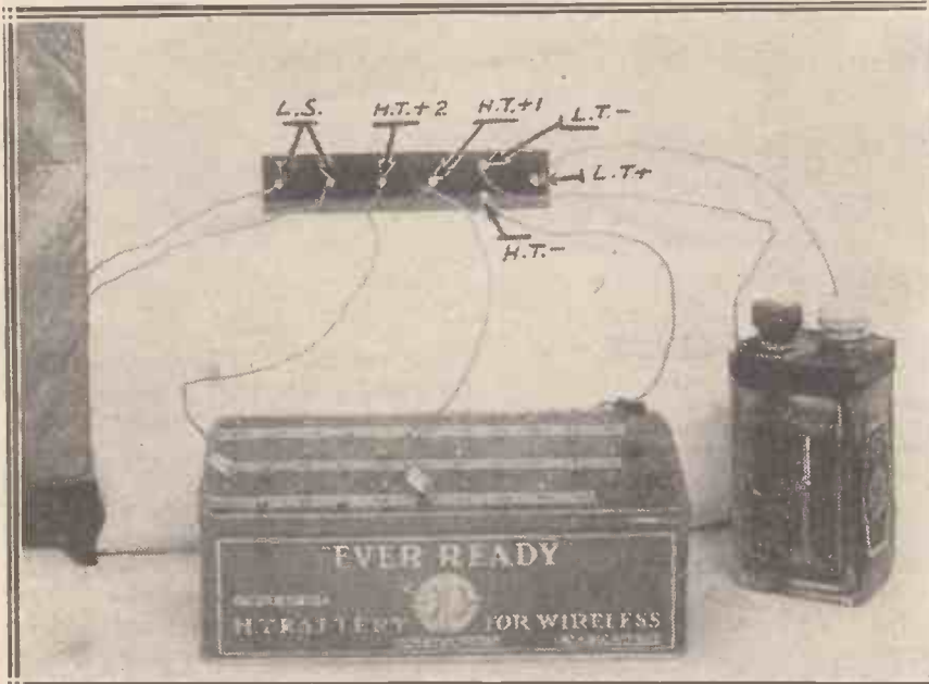
This view of the battery connections from the batteries to the special plug shows the latter as you would see it if it were plugged in place on the terminal strip. It is immaterial which way round the loud-speaker leads are joined.
