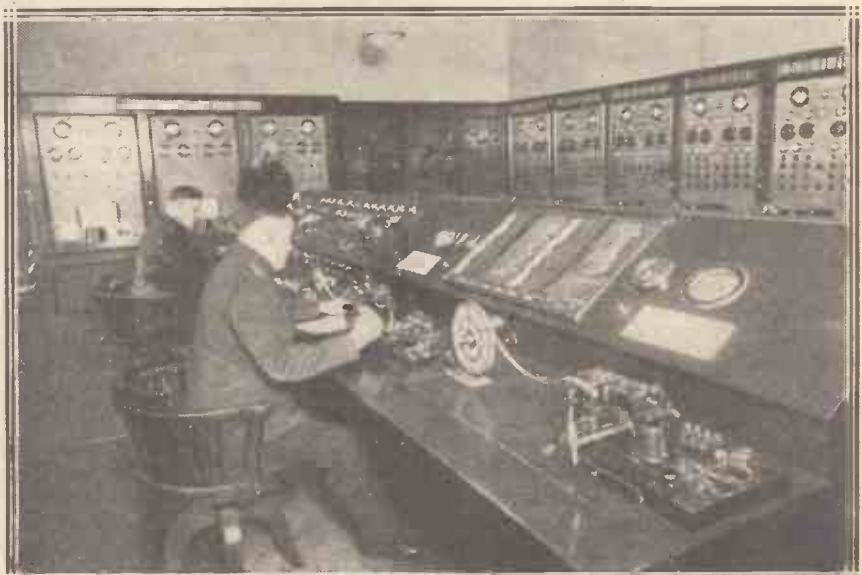
Some of the modern radio apparatus that Siemens and Halske have installed at the Berlin Central Fire Brigade Station.
