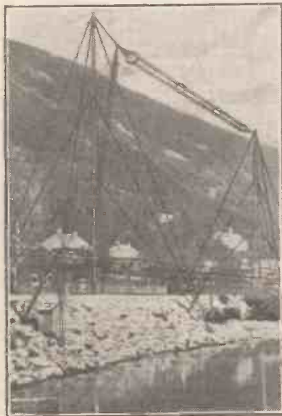
A relay station placed in a valley in order to pass on programmes from a shielded station.
