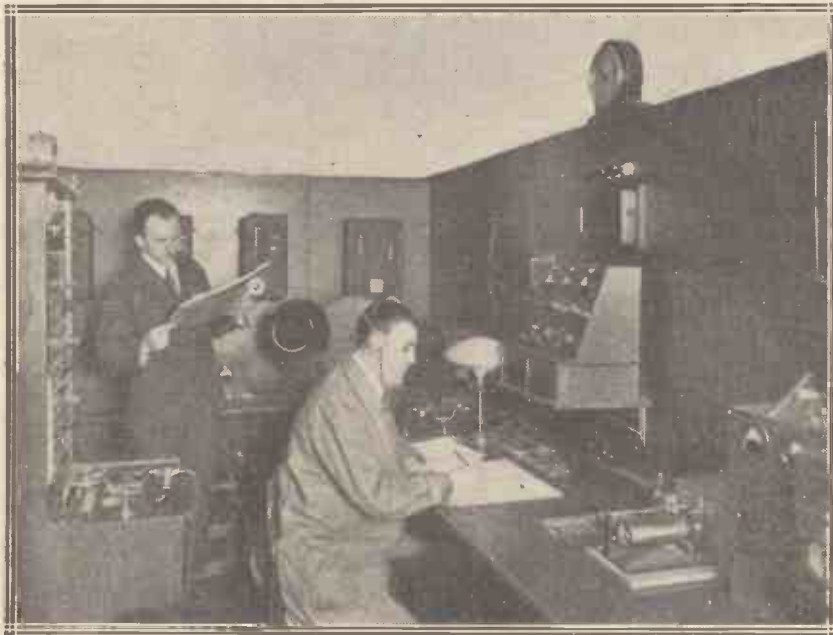
This is the control-room of the Oslo station. Oslo uses the comparatively low power of 1 kw., but is frequently heard in this country even on simple sets.
