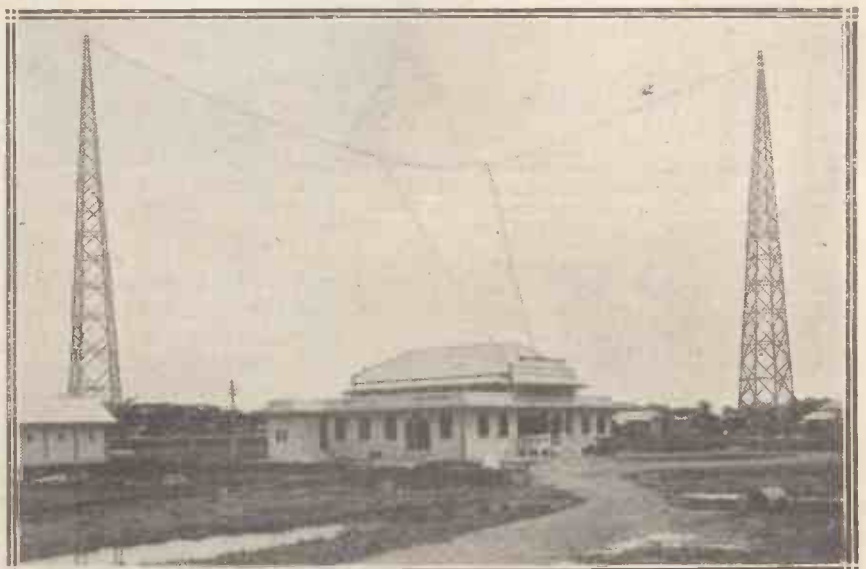
This is the short-wave station at Bangkok. The two masts each carry an aerial; the one for 14-metre and the other for 18-metre transmissions.
