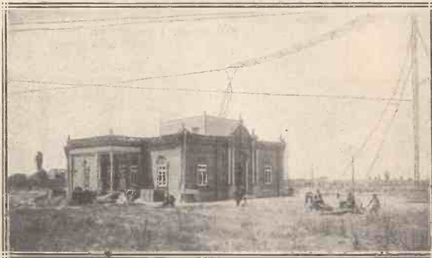
The new wireless station at Tabriz favours the cage type of aerial which is suspended from one main mast, as shown.
