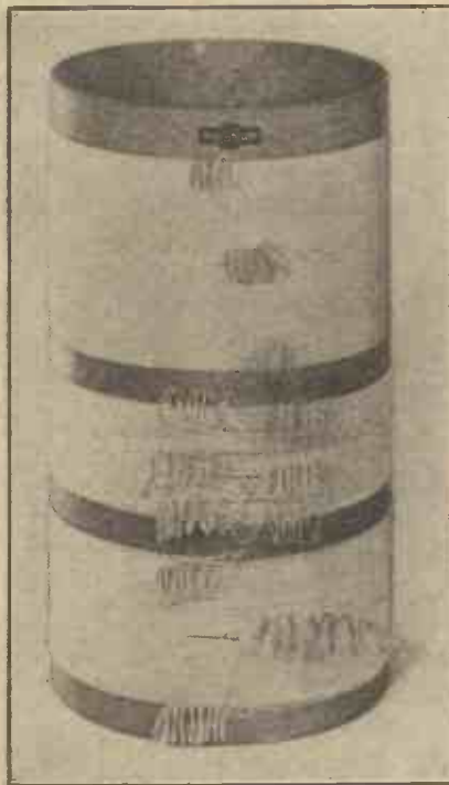
The specially designed coil used in the H.F. Unit.
