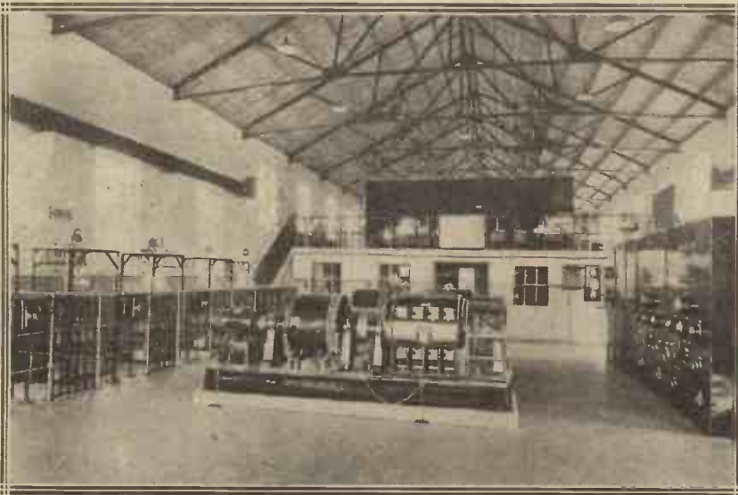
A view of the Marconi Beam transmitting station at Dorchester. Seven Beam transmitters are installed on the raised platform shown at the back of the picture.
