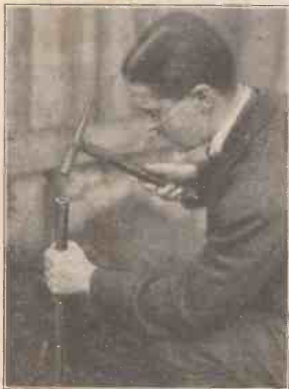
Now is the time to look to your earth connection, a point in your equipment upon which much depends. An earth tube of the type shown in this photo is a good device for all-round efficiency. It should be well driven into moist ground.
