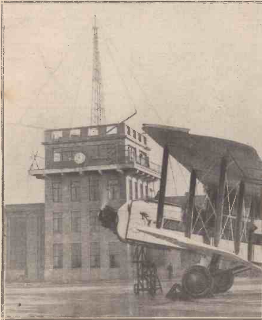
One of the features of the great new Croydon aerodrome building assemblies is the wonderful modern radio equipment. On the control tower can be seen the aeriavls used for direction finding, but the transmitters are at Mitcham. An intricate system of remote control is utilised.
