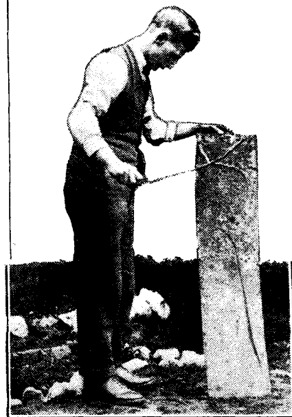
One of the earthing-plates mentioned in this article.
