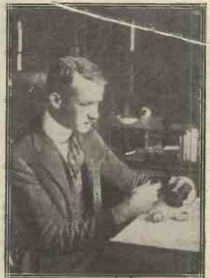
An assistant at the U.S. Bureau of Standards examining the small quartz crystal used for controlling a transmitter.
