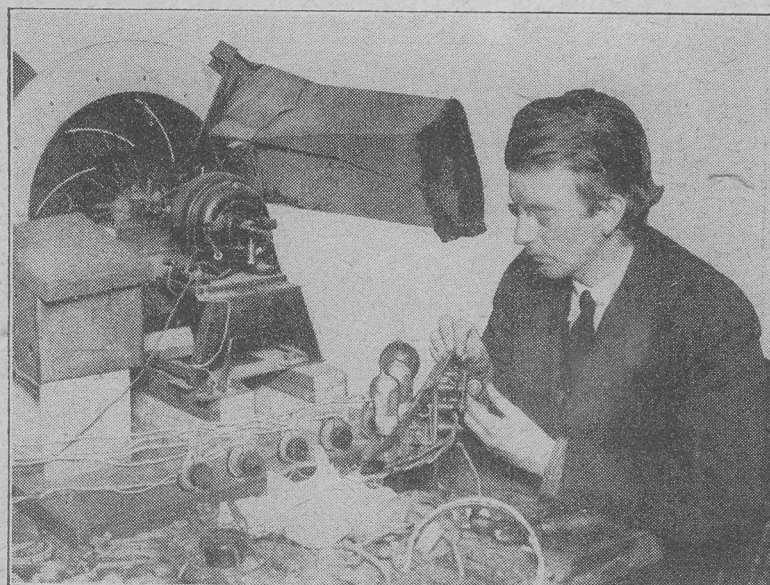
Mr. J. L. Baird and the apparatus with which he claims to have accomplished television.
