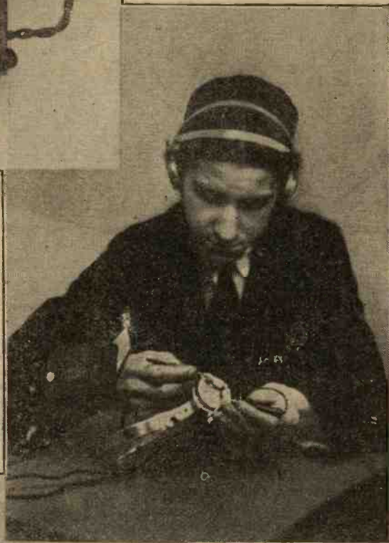
Telephone windings are easily tested.
