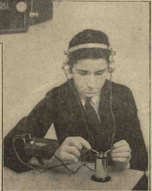
Testing transformer windings.
