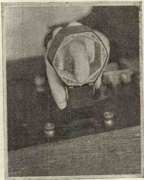
Place the coil in its socket this way, and . . .
