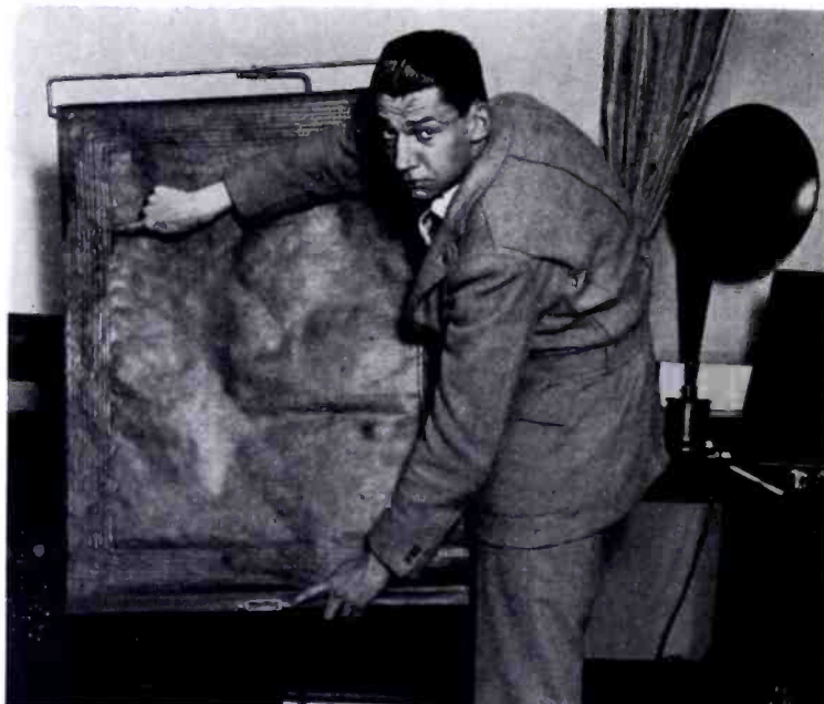
This novel indoor loop antenna consists of wire sewn to an ordinary window shade. Designed by W. H. Bullock
