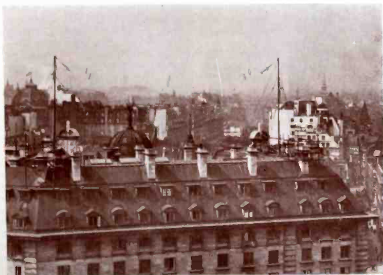
Antenna system of the British Broadcasting Company's 2LO station which operates on 369 meters
