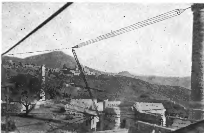
Six-wire cage antenna of BX amateur station. The illustration gives a good view of the surrounding country, including the location of the remote-controlled 20-watt transmitter
