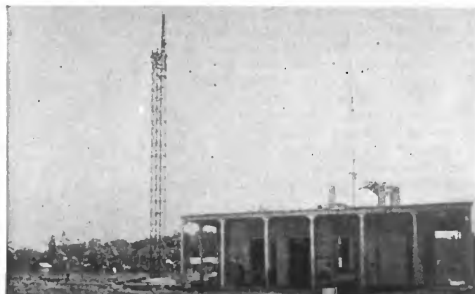
The Cayenne station, showing the mast, and the deep-poricoed operating building, which contains shower baths as well as radio apparatus
