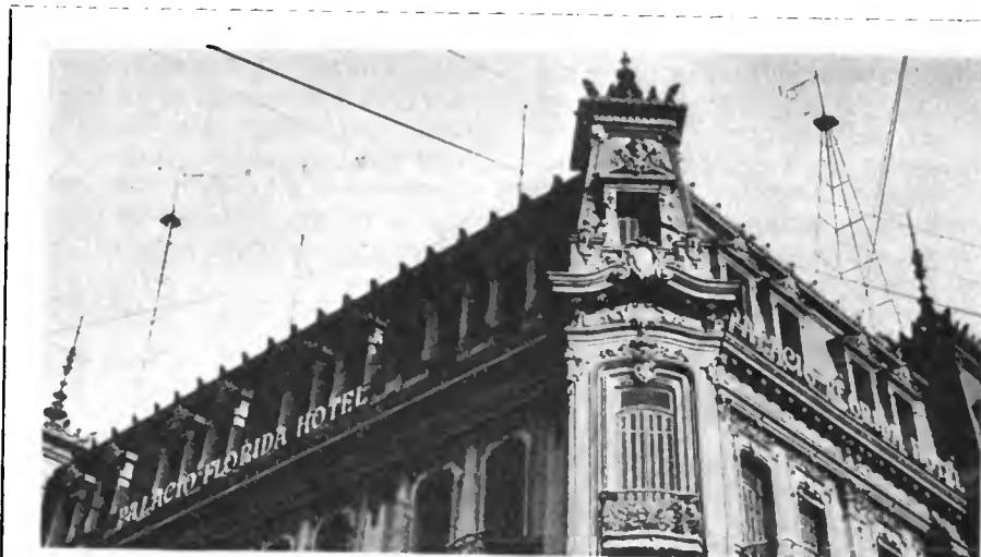
Montevideo and its neighbors now get daily thrills from the new broadcasting station erected on the roof of its leading hotel
