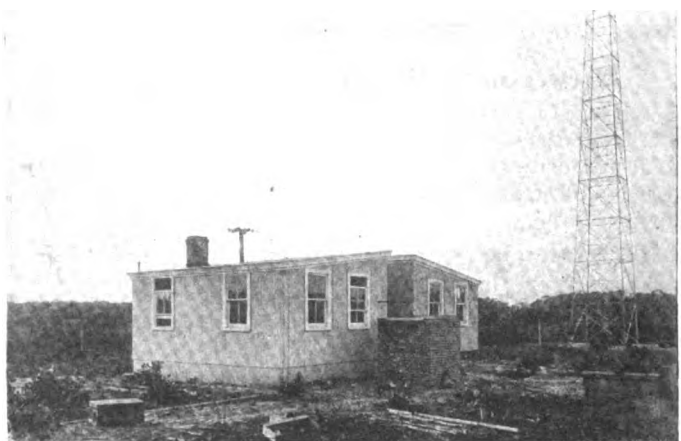
Easthampton Radio Station in course of construction
