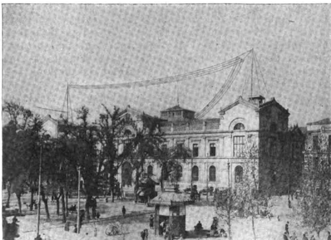
Distorted L antenna 35 meters high and 60 meters long, running east to west, which is unfavorable for northern reception
