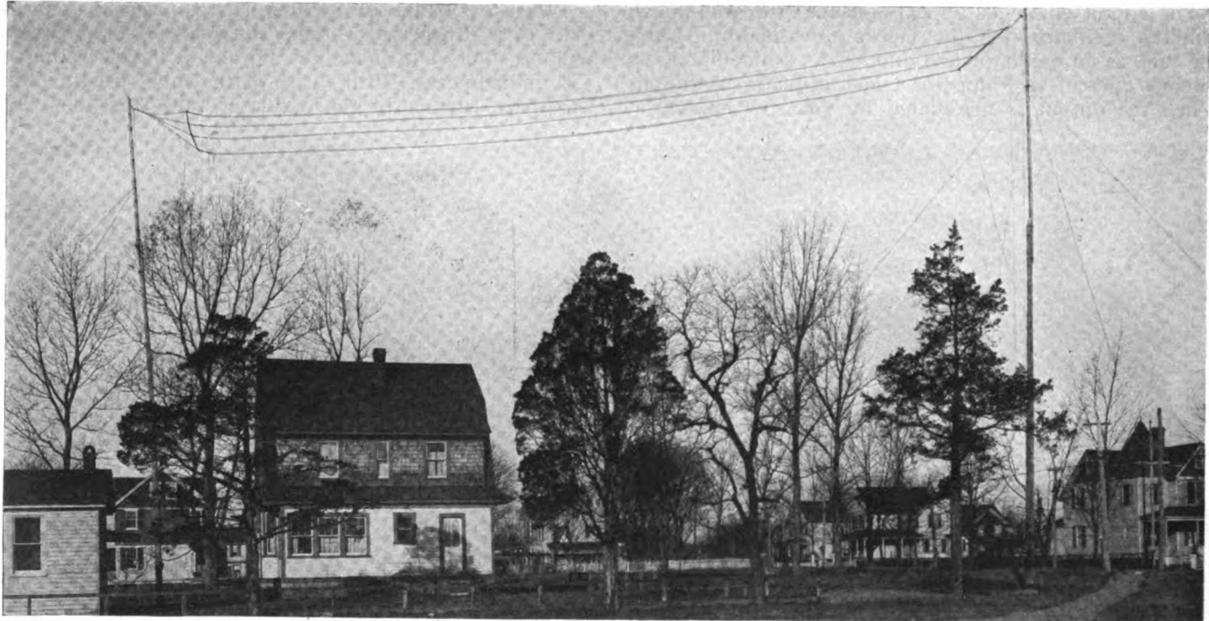
Antenna and counterpoise ground system at 2ZL. The antenna is 120 ft. long between spreaders. The counterpoise ground is used because of the dry sandy soil. It consists of 7 No. 21 copper wires, directly under the antenna, also on 15 ft. spreaders. Both spreaders and wires are insulated from ground
