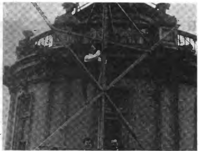
Keystone Erecting the receiving loop on the N. Y. Times Bldg., with which it was hoped to receive radiophone messages from warships entering the harbor
