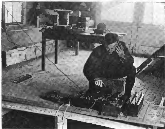
Receiving apparatus used in telephoning and telegraphing by means of bare wire laid in water
