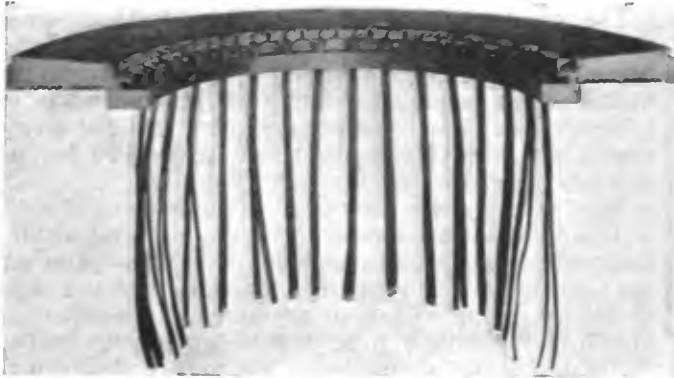
Figure 7—A section of the armature
