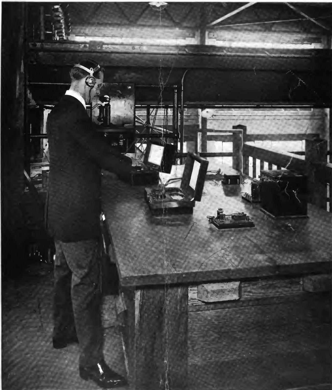
The Supervisor and His Instruments at a Trans-Atlantic Radio Transmitting Station
