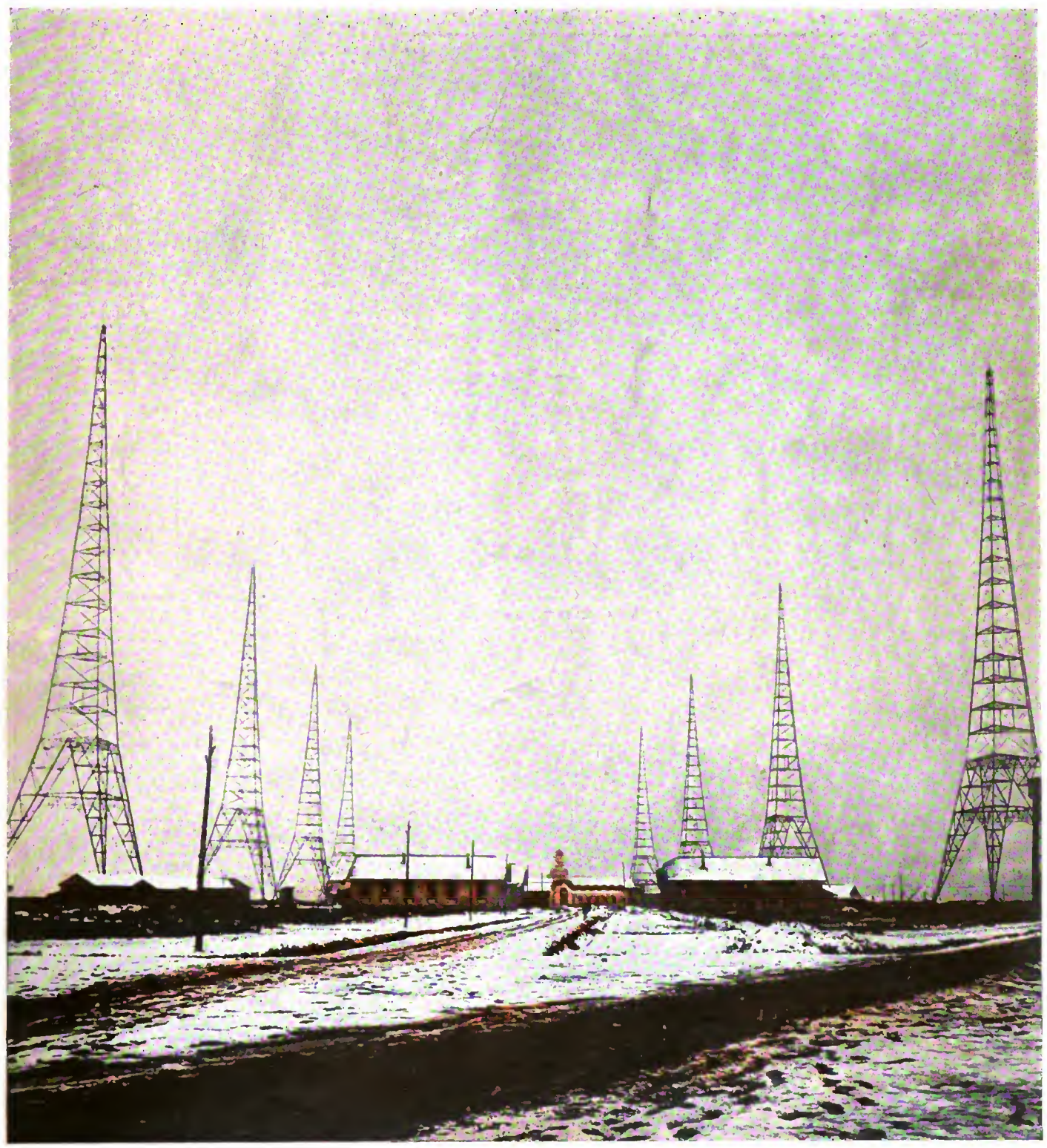
The Lafayette Trans-oceanic Station Near Bordeaux, France, Showing Eight Towers, Each 825 Feet High
