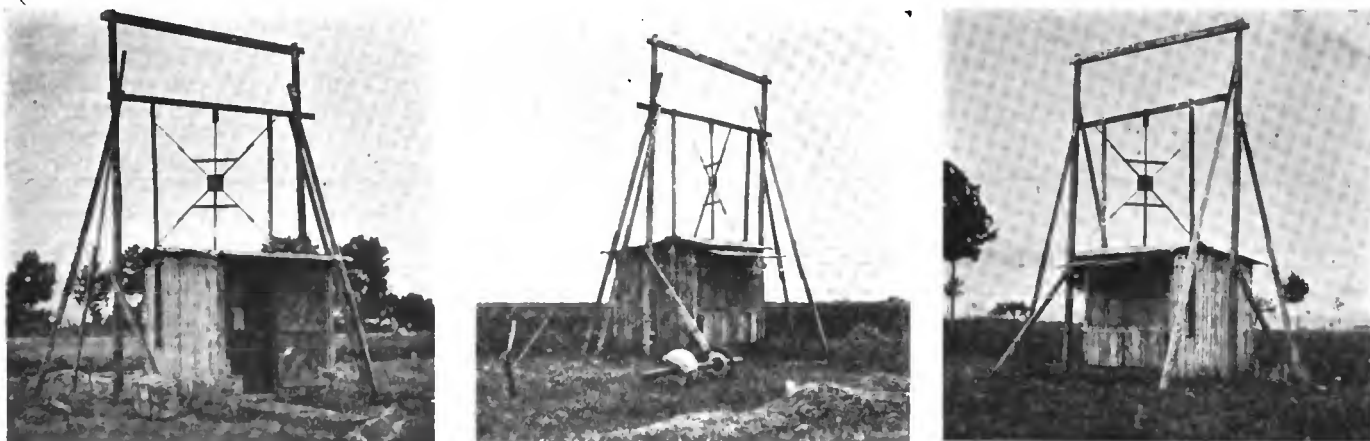
Radio goniometric stations on Toul front provided with small loops of American design
