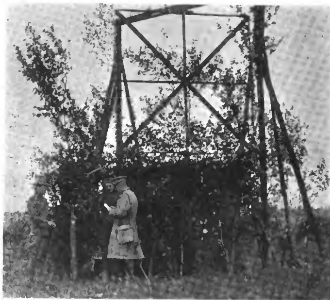
Radio division officer inspecting a camouflaged goniometric station on the Toul front
