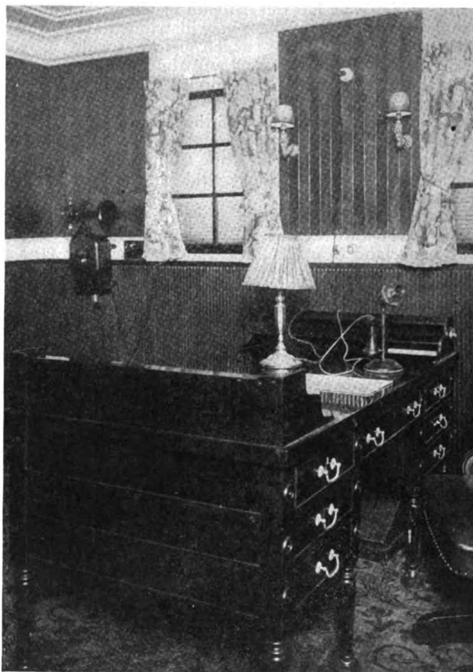
Telephone equipment installed in the President's room on board the steamship George Washington
