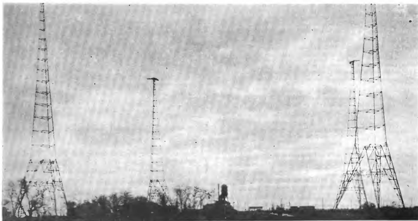
The four towers of Annapolis forming a square within which the aerial wires are strung. A feature of the gigantic antenna is the provision for melting ice from the wires by current supplied from the 400-kw. generators
