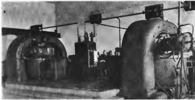
The two arc converter machines installed in Annapolis station, showing the benchboards from which the engineer controls the whole station
