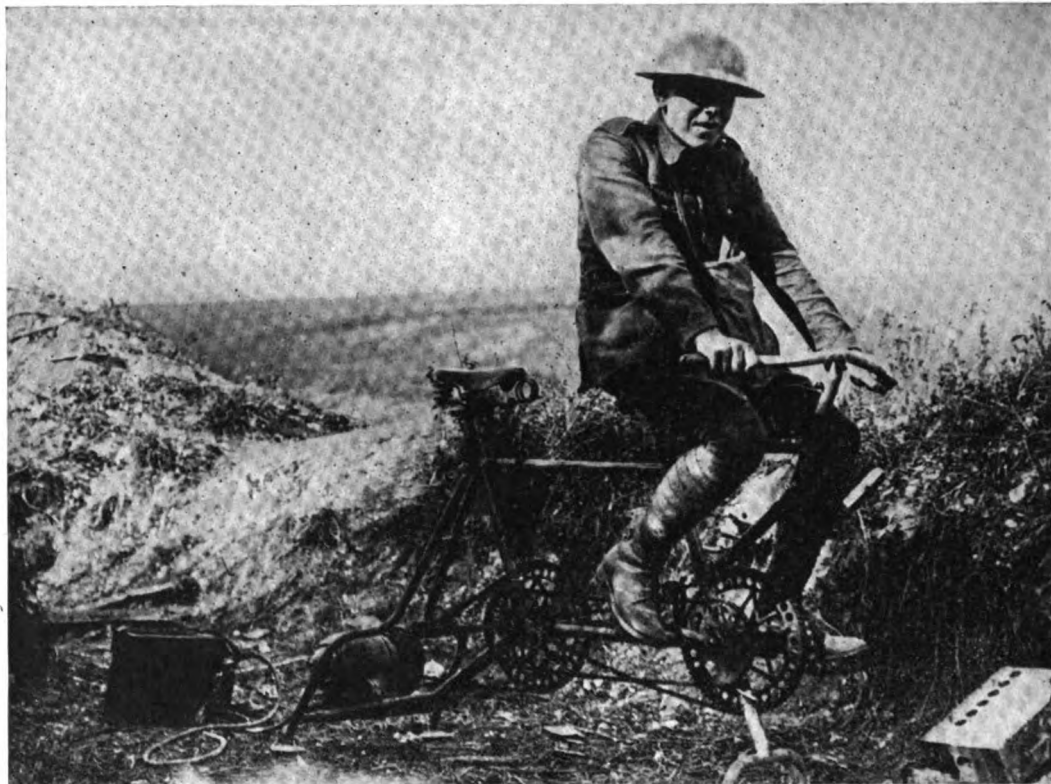
British Off. Photo Apparatus captured by the British from the Hun who used it to generate electricity for their wireless stations
