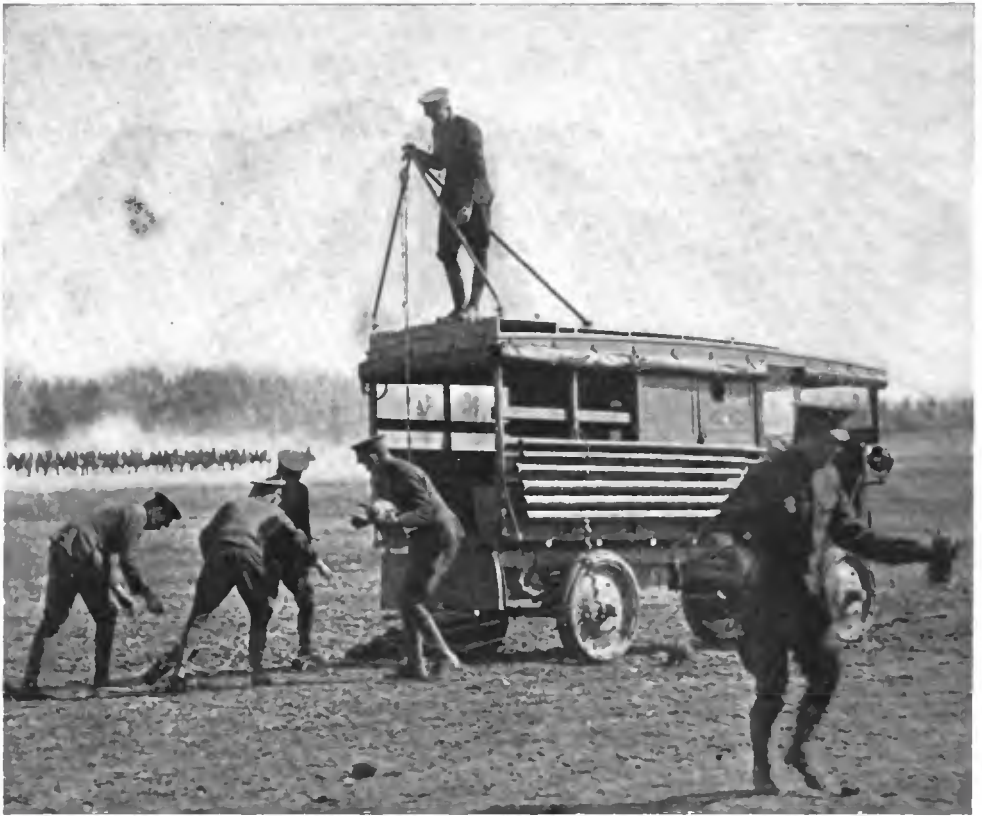
Members of U. S. Signal Corps attaching support for wireless pole to the new auto radio truck
