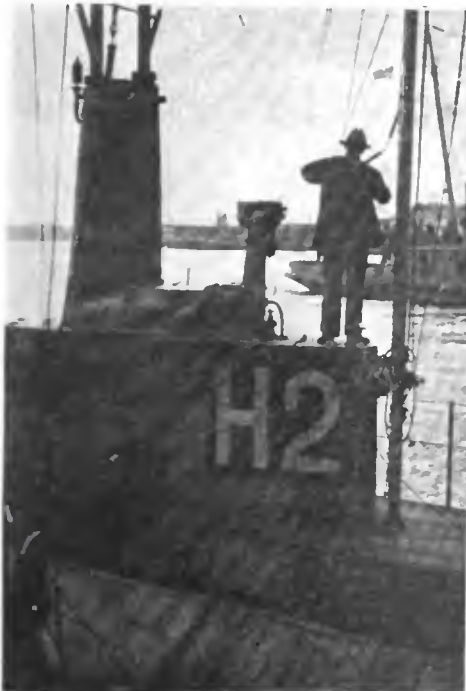
The wireless mast and deck insulator are just at the point of the shears
