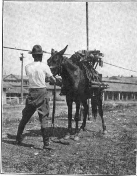
The generator and frame of the apparatus on a pack mule
