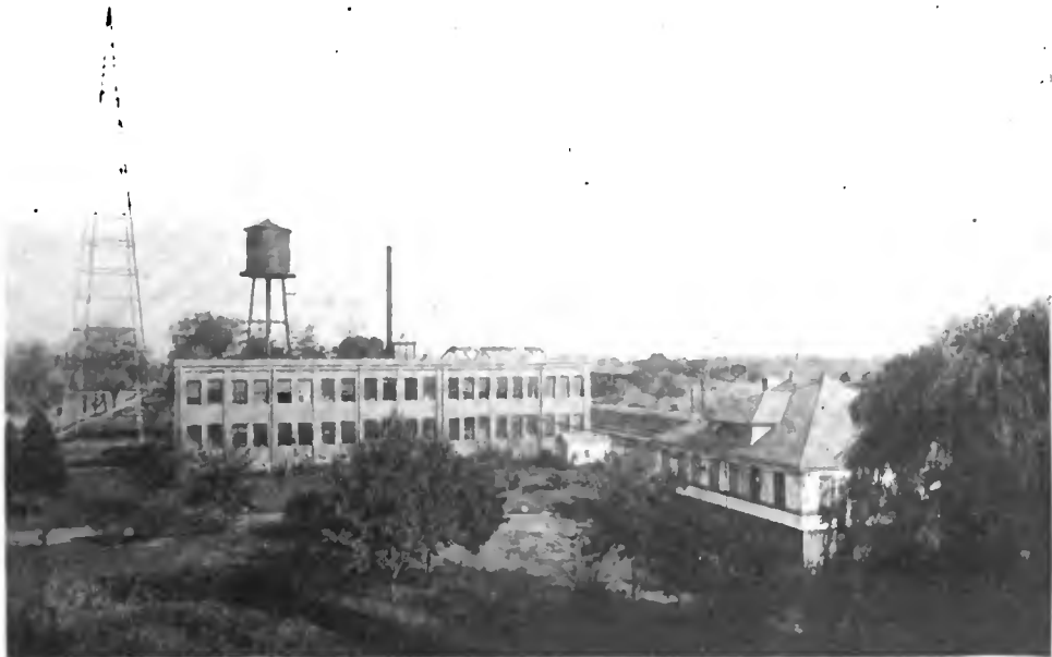
A view of the Marconi plant at Aldene, N. J., taken from the elevated tracks of the railroad, showing the west side of the factory building, a portion of the laboratory, oil house, tank for sprinkler system, one of the wireless towers and the surrounding grounds
