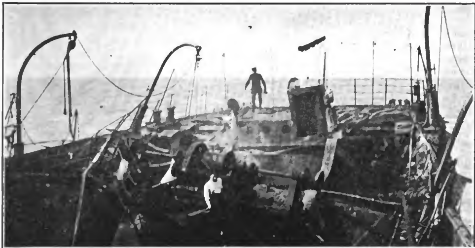
After the explosion
