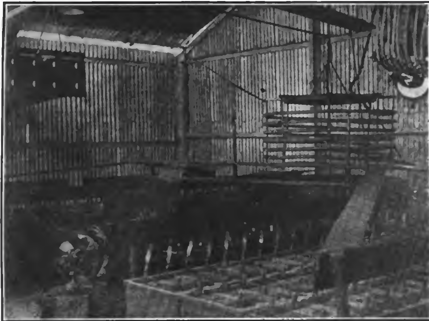
The condenser room of the 150 k.w. station at Manaus, from whence the survey party of the Brazil-Bolivia Commission received its longitude signals on a portable set erected each night in the depths of the jungle
