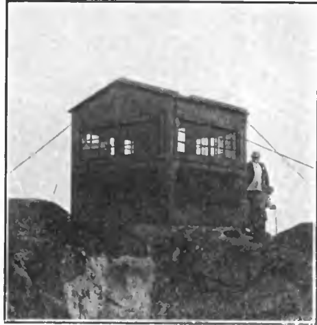
The forest-fire warden's house which provided protection for the author of this article and his companion during a storm
