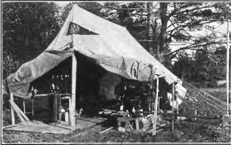
Above, the military headquarters' wireless station, giving a glimpse of the condenser rack and the 8 h. p. Fairbanks-Morse engine used for generating power for the 2 k.w. set loaned by the Marconi Company. Both engine and wireless apparatus were donated by the respective makers in the interests of patriotism. In center, Officer of the Day on inspection rounds
