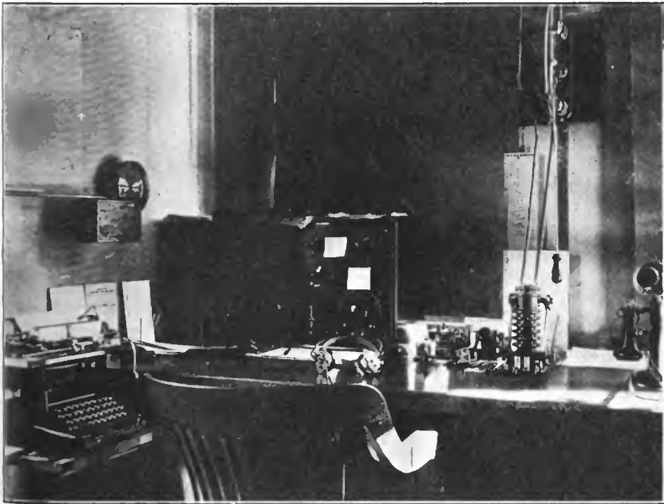
The operating table is connected with the engine room by a thin wire rope running on pulleys and attached to the high tension magneto, enabling the operator to start the engine on a retarded spark without moving from his place
