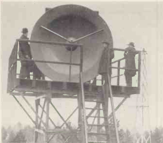
Terminal tower and antenna at Lymgne in the s.h.f. link with St. Inglevert, France.
