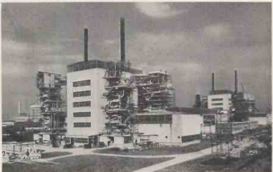
General view of Calder "A" showing the turbine hall flanked at each side by a reactor building—the heat exchangers are located at the corners of the reactor building. Behind Calder "A" and to the extreme left can be seen the Windscale factory.
