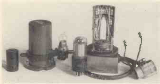
Photo-multiplier cell and lamphouse assembly
