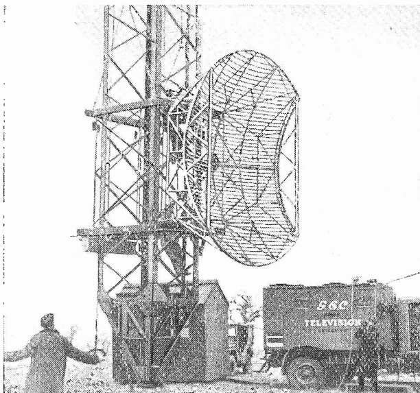
Fig. 1. The temporary masts on which the paraboloid aerial can be raised or lowered
