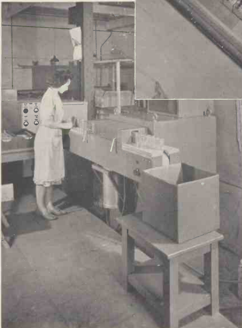
Fig. 1 (above). Overall arrangement of the soldering conveyor assembly, showing the oil-filled tank condenser projecting below the conveyor housing.
