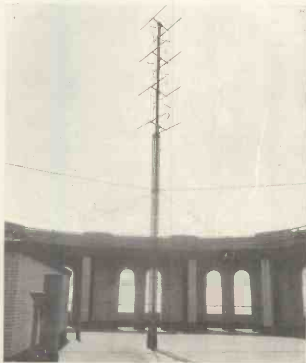
The ultra-short wave aerial on top of an office building in New York.
