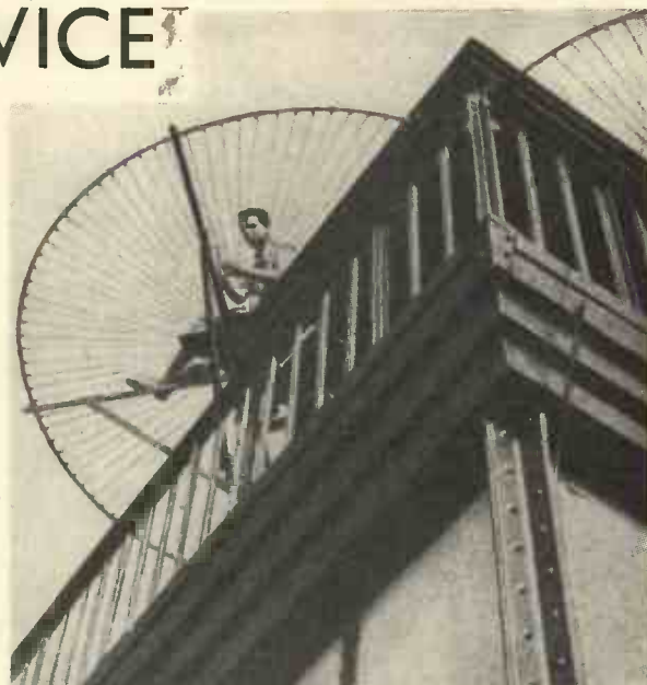
The ultra-short wave aerials on top of the Berlin Funkturm tower.
