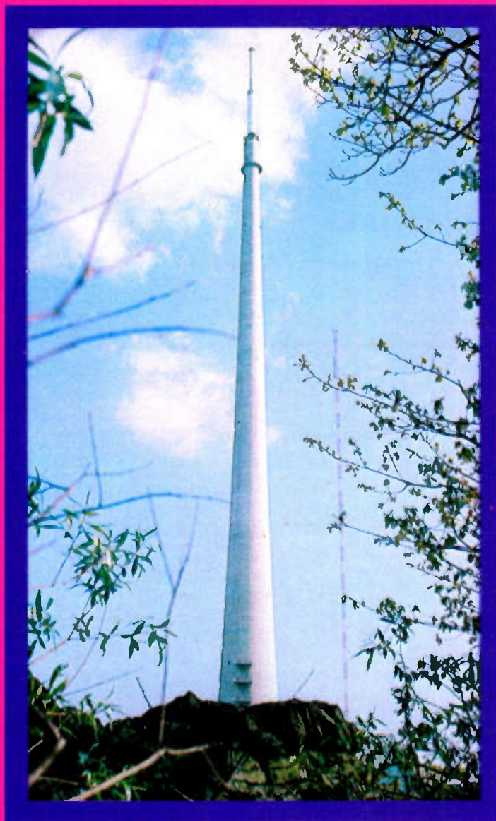
The IBA's 1,080 ft aerial tower at Emley Moor in Yorkshire is the first self-supporting concrete tower ever to be built for television broadcasting in the United Kingdom. An IBA film, Tale of a Tower , shows its construction and explains some basic facts about television broadcasting.
