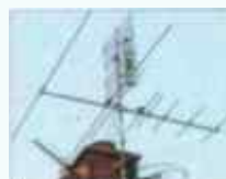
Chimney-mounted antenna system used by Martin Dale in Stockport. The lower array covers all v.h.f. frequencies in Bands I, II and III. The u.h.f. array is a wideband grid.
