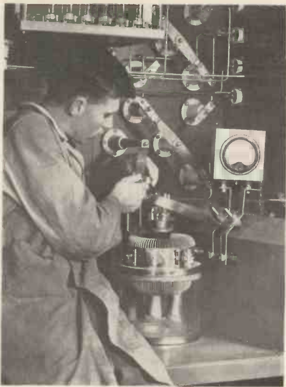
RADIO NEW ZEALAND. Installing one of the high-power valves at the new short wave transmitter at Titahi Bay, Wellington, N.Z.
