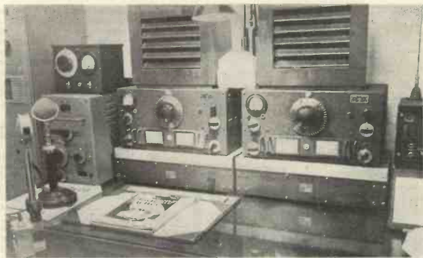
G2AMJ, Willerby, East Yorks., is a "28 mc only" operator, and was featured in the "Other Man's Station" series in the April issue of our parent Short Wave Magazine . This is a view of the receiving position, with two HRO's used together.
