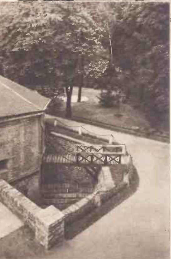
The Luxembourg studio block, situated in the middle of a park, showing part of the old fort and drawbridge
