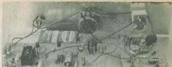
A view showing the front panel components from the rear
