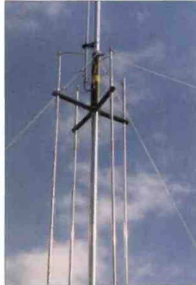
Fig. 1: David guyed the Titan antenna as it was only a temporary installation.
