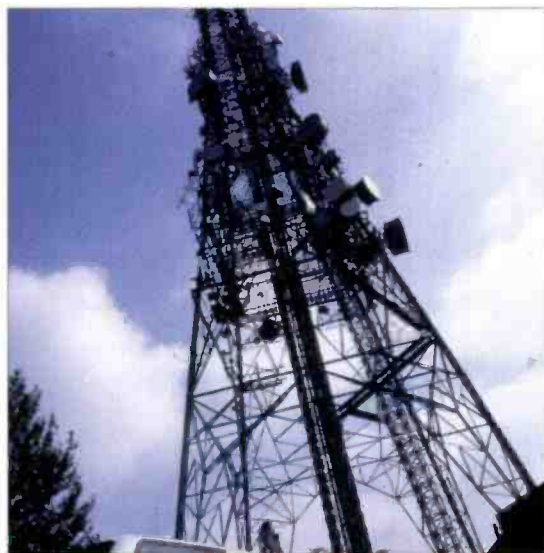
One of the NTL's transmitter masts situated in Croydon in South East London.
