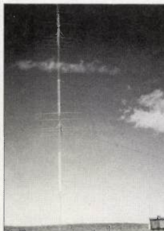
Fig. 4: This 200ft tower holds a 'six over six' for 14MHz and is John's largest tower.
