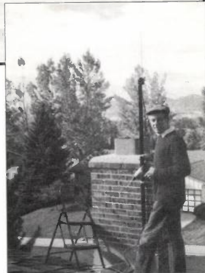
Ed WT3U installs a new 144MHz vertical antenna on his house chimney.
