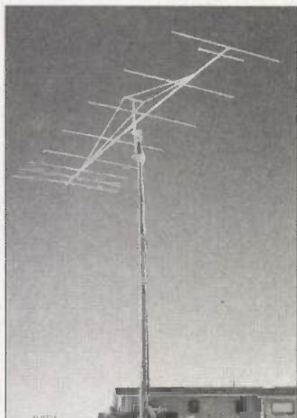
Fig. 3: The lowest antenna on W0UN's 60 acres is his eight-element single band array for 21MHz.
