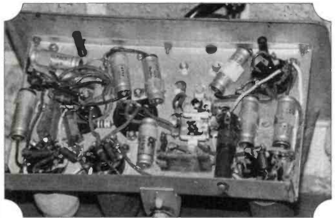
Fig. 2: Receiver section of the 18 set, removed from case for servicing, showing metal cased tubular capacitors (see text).
