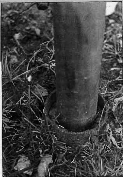
Sand should be packed into the space. It gives under strain, but holds the base section in place.
